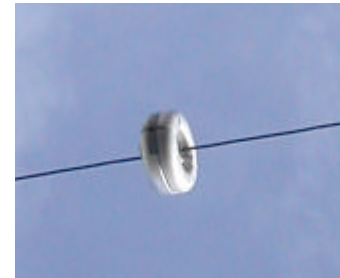
Aerial Conductor Installation
